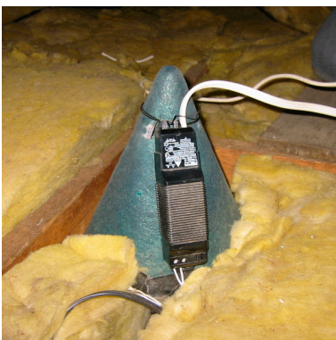
Mitt install from below ceiling
