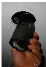
Mitt install from below ceiling
