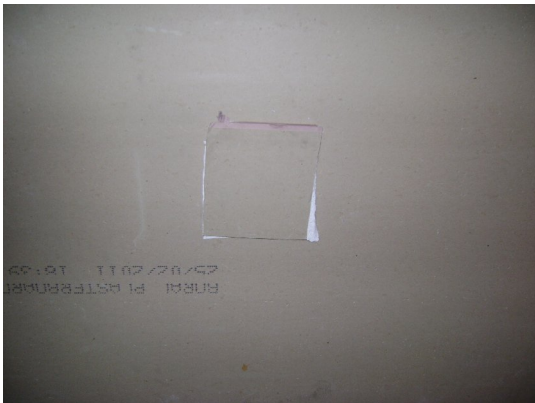
Figure 2.4: 16mm plasterboard fill installation, from receiving and source rooms respectively
