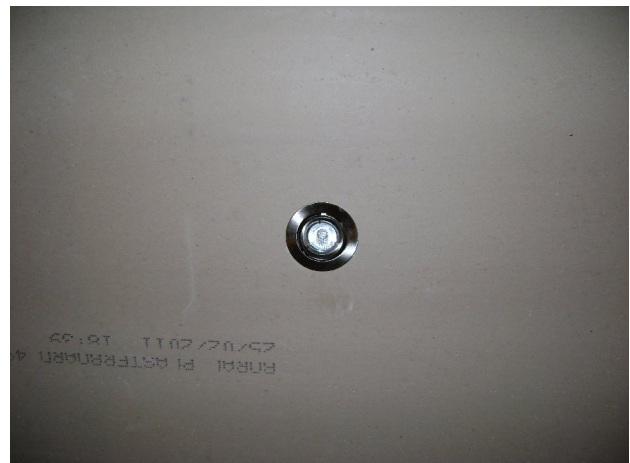
Figure 2.2: Downlight installation in plasterboard (from receiving chamber)
